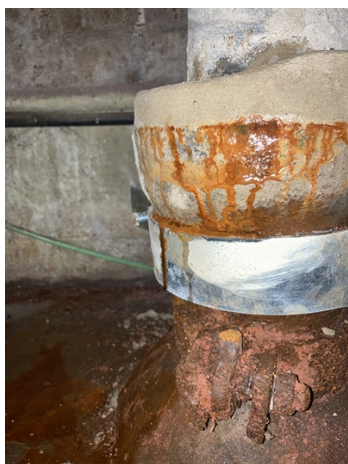
Leak through the hydraulic cement
