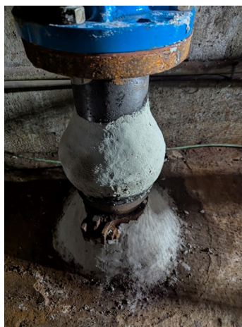
Belzona 4141 to smooth out transition area
