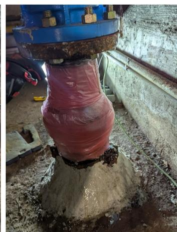
Full system wrapped and seal with Belzona SWII
