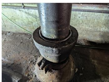
Hydraulic cement removed and pipe cleaned with power tools to bare metal
