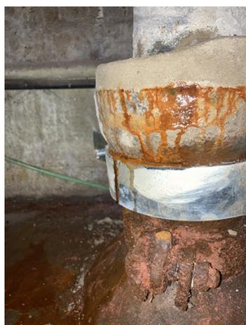
Leak through the hydraulic cement
