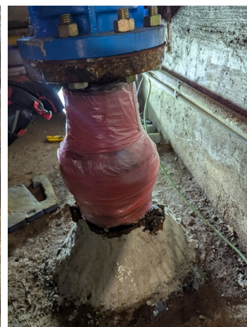
Full system wrapped and seal with Belzona SWII
