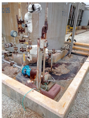
Acid containment with damage in concrete before application
