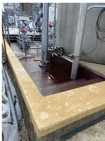
Belzona 4311 applied into containment
