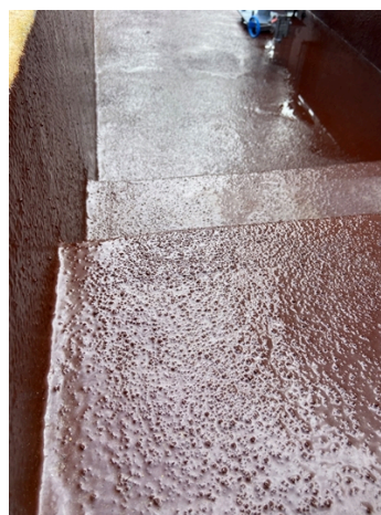
Close up on coating with non skid aggregate
