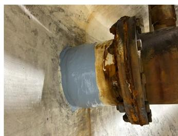
Full repaired section protected with Belzona 1341N
