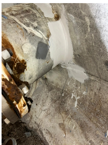
Cold bonding repair completed and through wall defect sealed
