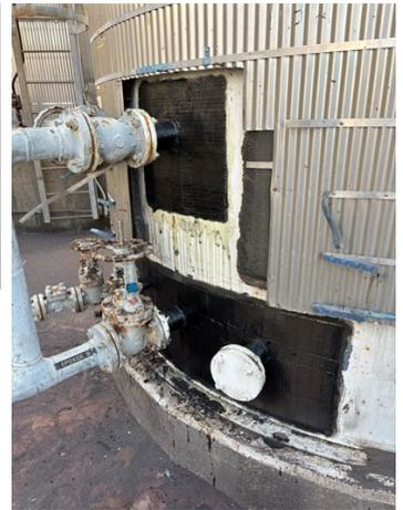
Insulation removed and can see the pitting / external corrosion on the nozzles
