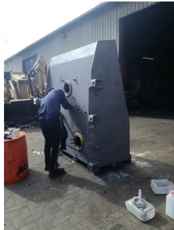
First coat with Belzona 5811
