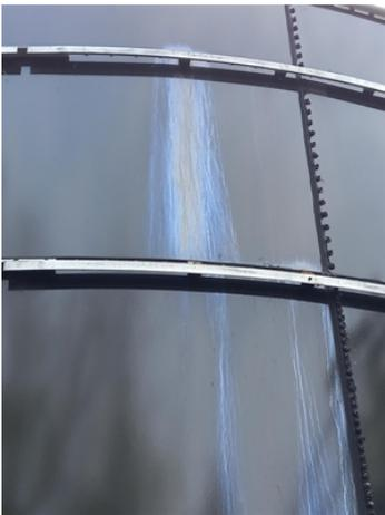
Leaks showing throughwall on large settlement tank
