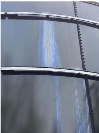
Leaks showing throughwall on large settlement tank
