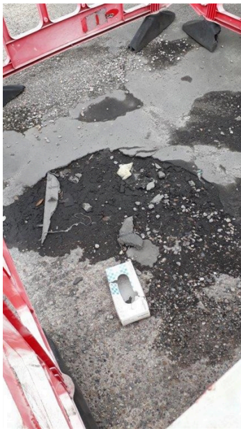
Broken floor with large holes and cracks due to impact
