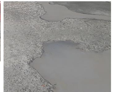
Broken floor with large holes and cracks due to impact
