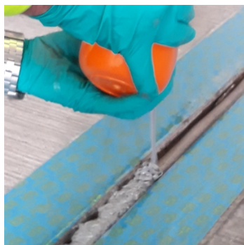
Joint prepared and 4521 being applied
