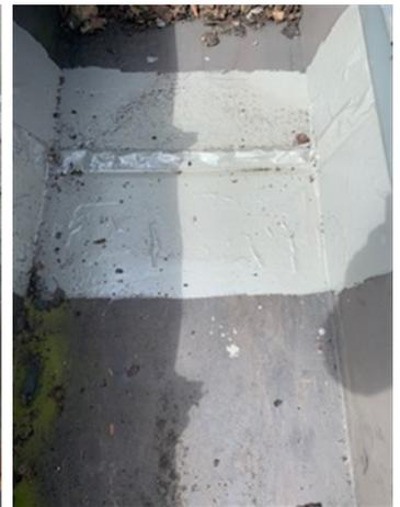
Areas of probable leaks were identified on external inspection of the high bay
