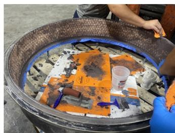
Belzona 1812 Grout
