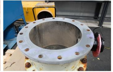
The cooling spools have been reprofiled and repaired, ready to be reinstated
