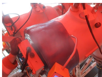
Completed SF6-FIX application with final layer of Belzona 7311
