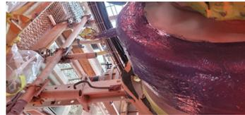
First layer using Belzona 7311 and 9341 open mesh reinforcement fabric over the breather membrane and breather tube.
