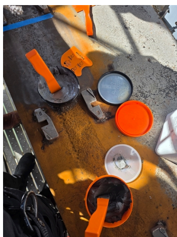
Condition of the rail bed flange before surface preparation
