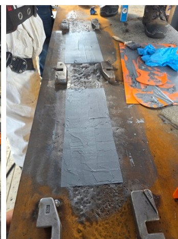
Application of Belzona 1121 completed in two sections
