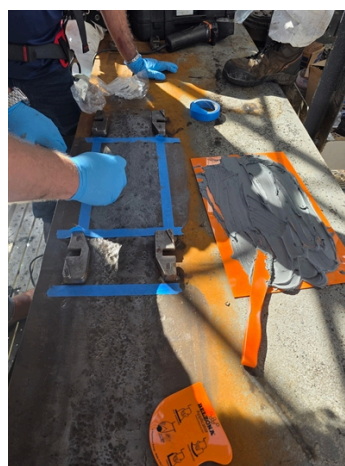
Belzona 1121 being applied
