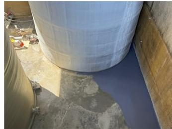
Application of Belzona 4311
