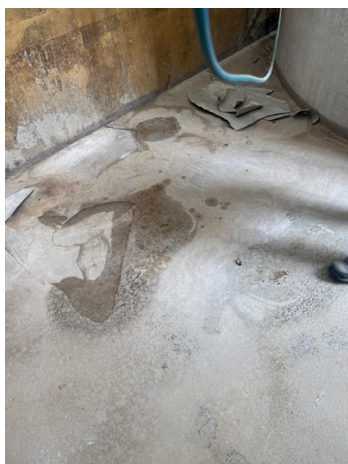
Failed previous coating
