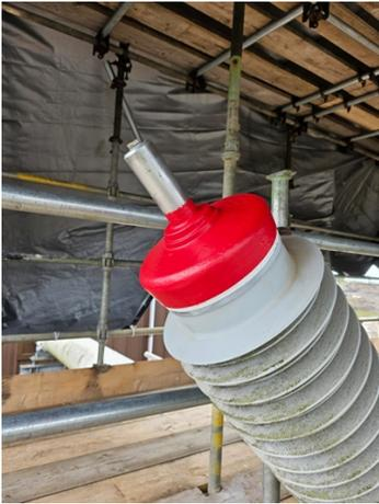
Existing coating this was removed & the surface prepared.
