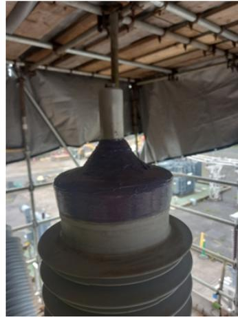
Belzona 7311 built up & Belzona 9341 reinforcement added.
