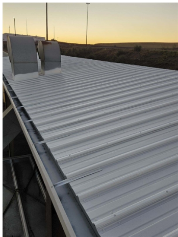
Belzona 3111 applied on 100% of roof with mesh installed on all seams fully reinforced.
