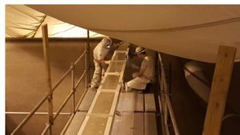
Application of Belzona 5811DW2 by brush to the legs of the clarifier
