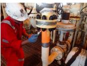
Corroded flanges in the oilfields The technician applied the first The second coat of Belzona coat of Belzona 3412 to protect 3412 was applied on the the flange.
