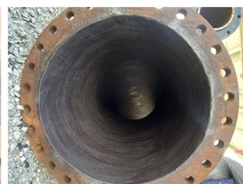
Dredge completely coated with Belzona 1814.
