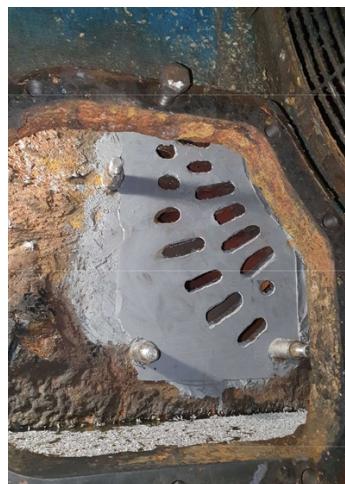
Former plate applied to defective area and Belzona 1161 allowed to cure
