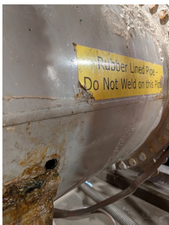
A hole in a pipe before the application.
