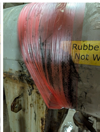
Strengthening the repair with Super Wrap II with Belzona 1984
