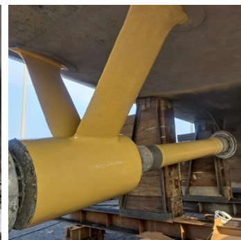
Application of second coat of Belzona 5821
