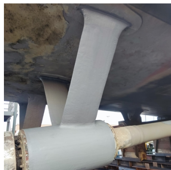
Belzona 1111 (Super Metal) was used to rebuild and fair the pitting damage on the substrate
