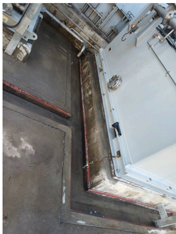
Cleaning in progress. Belzona 9111 degreaser, concrete cleaner & a water based detergent were used and then high pressure washed with clean water.
