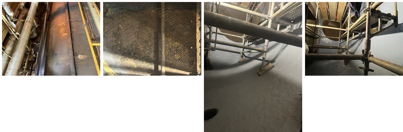
New metal work installed on condenser Existing internal metal before preparing for coating Substrate after applying Belzona 1121 Substrate after applying Belzona 5821
