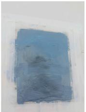
To strengthen the repair area, UW-Metal) was applied before plate bonding method. proceeding with plate bonding.
