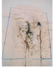
A leak in the wall of the customer's fire water tank created a hole and disrupted operations.
