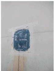
Following cleaning, the substrate was grit-blasted, and Belzona 1161 (Super Belzona 9611 (ES-Metal) was applied to effectively seal the leak.
