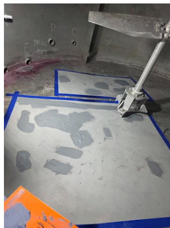
Abrasive Blast prep (SSPC-SP10)
