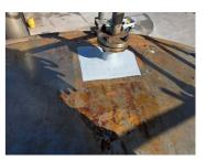
Belzona 9611 applied to seal the vapors, and a sparkless grinder used for surface prep (SSPC-SP11)
