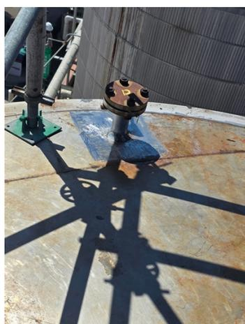
Belzona 9611 applied to seal the vapors, and a sparkless grinder used for surface prep (SSPC-SP11)
