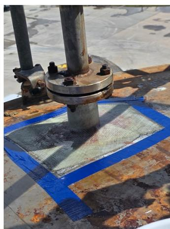
Belzona 4181 resin wet out into Belzona 9371 fiberglass reinforcement mesh to composite wrap the nozzle
