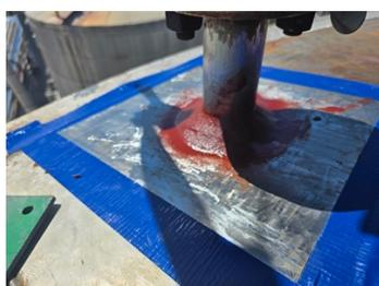
Belzona 4181 mortar applied around the neck to create a smooth chamfer for the composite wrap
