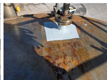
Final image with Belzona 5721 top coat applied
