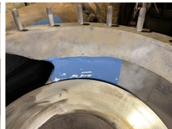
2nd coat of Belzona 1321 Ceramic S Metal applied
