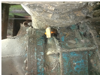
Temporary leak fix
