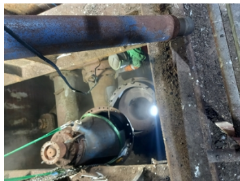
Casing accessed during shutdown & grit blasting underway
