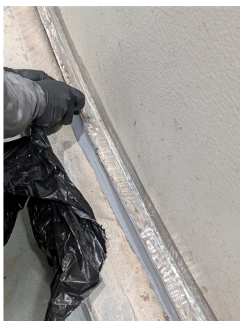
Stemming the leak with Belzona 1161
