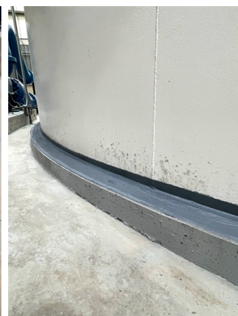
After application of two coats of Belzona 3111 with mesh.
