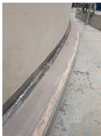
Sealing the perimeter with Belzona 4111
