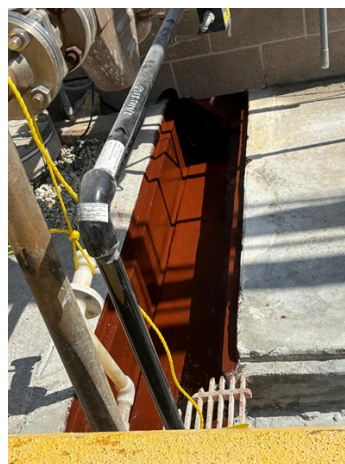
Belzona 4311 application complete
