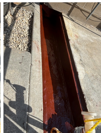
Belzona 4311 application complete
