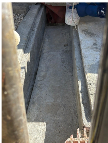
Image of the relatively new poured concrete drain area, before the coating work began
