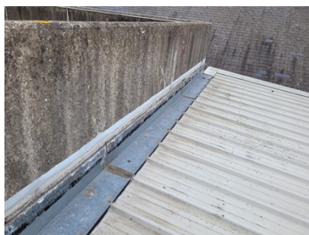
Flashing not sealing between concrete face and over existing roof.
