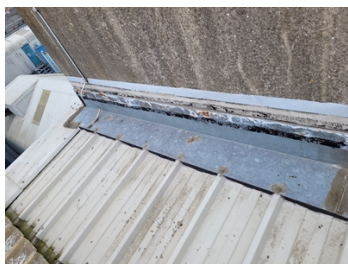
Original problem area showing leaking flashing baffle.
