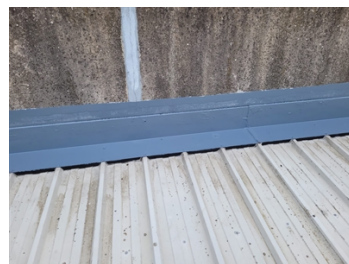
Face on view of the complete Belzona 3131 system repair.
