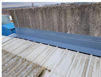
Completed repair using the Belzona 3131 system.
