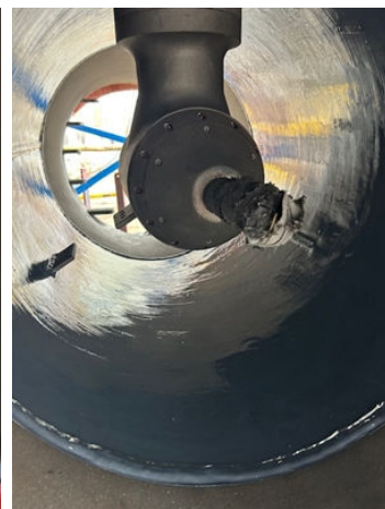
Job completed after 2nd coat of Belzona 1321 coating.
