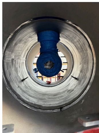
Belzona 1311 used to fill all pitting in tunnel.
