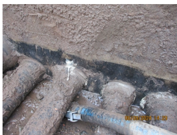
Close up showing leak path
