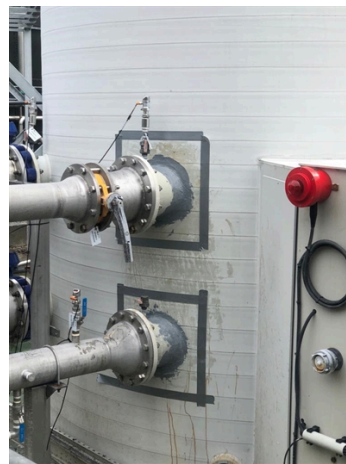
Belzona 1221 applied
