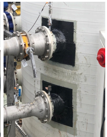
Belzona SuperWrap II system applied
