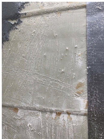
Surface preparation on the plastic tank
