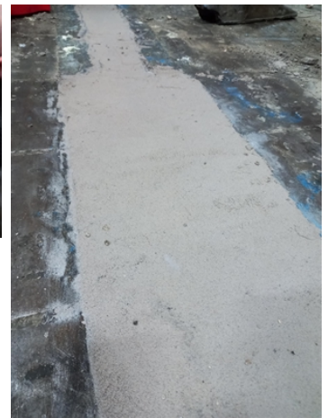
Completed application using Belzona 4131
