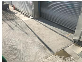
Completed repair using Belzona 4131
