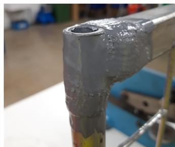
Belzona repair using Belzona 1111 and reinforcing sheet
