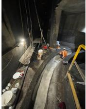
The channel was rebuilt using Belzona 4151 (Magma Quartz Resins) and locally sourced fine the fabric backing was quartz sand and then lined with removed, and the area was alumina tiles using Belzona 1321 (Ceramic S-Metal) as the adhesive.
