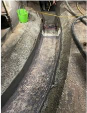
Once the grouting was complete, a feather edge of Belzona 1812 (Ceramic Carbide FP) was applied to create a tiles and the channel, helping to prevent future buildup of beards.
