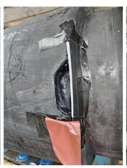
Dams were glued in place to retain the Belzona product during curing
