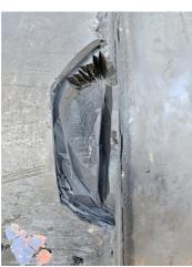
to remove any loose material, rotary burr before conditioning with GP Conditioner
