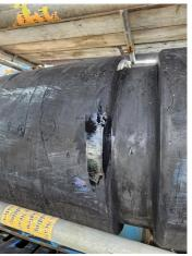
Belzona 2131 (D&A Fluid Elastomer) fluid was mixed with shredded rubber aggregate and applied into the repair areas
