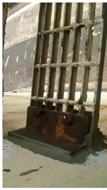
The grating stair was securely fixed to the tank shell.
