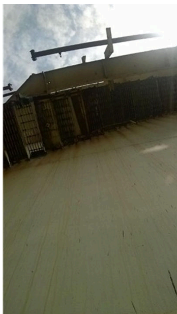
The staircase of the 79-meter-diameter crude oil storage tank was damaged.
