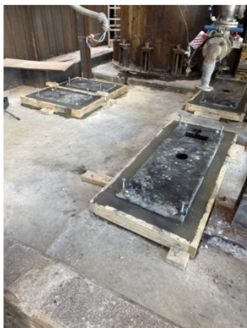
Contractors setting up the pump bases.
