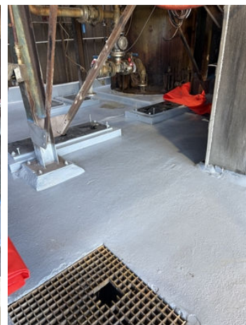
Containment after top coat of Belzona 5811.
