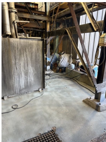
Containment after being cleaned and grit blasted.
