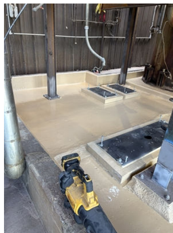
Containment during first coat of Belzona 5811.
