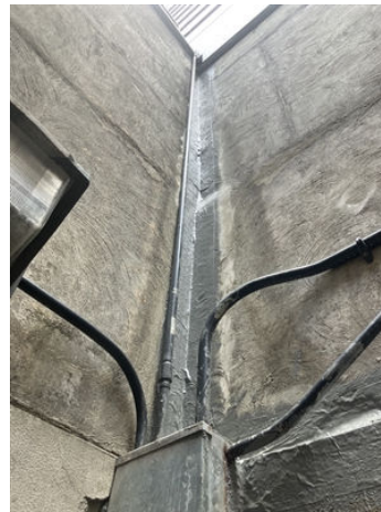
Close up on the vertical joint after the application was completed.
