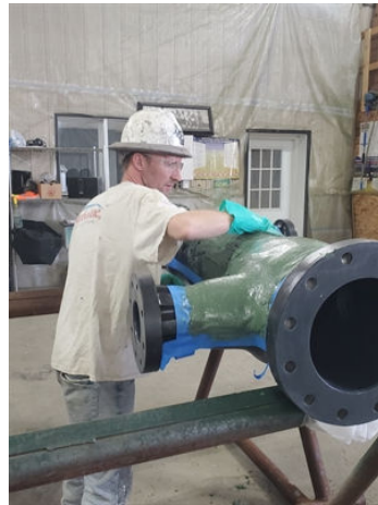
Closeup of contractor finishing up on a header.
