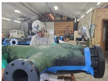
Smoothing out the Belzona 1813 on headers.
