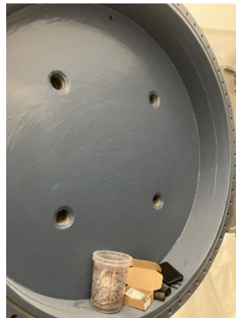
Belzona 1321 applied on the end cover
