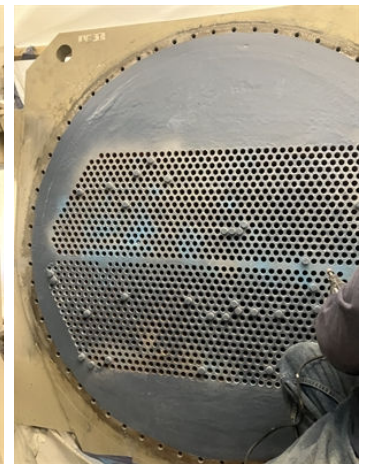
Belzona 1321 applied on the tube sheet
