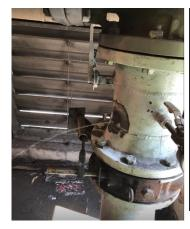
Assessing the situation before beginning. You can see the live the surface area using a MBX leak. This is where we came up Bristle Blaster to create a with the plan to stop the leak using Belzona 9611 and 1111 with reinforcement cloth.
