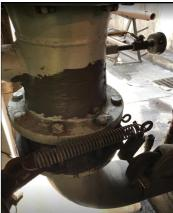
To complete the application, we applied Belzona 1111 to the surface area and to the reinforcement cloth and wrapped the entire spool.
