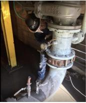
Next we cleaned and prepped profile for the Belzona to adhere to.
