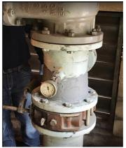
Once the preparation was completed we used Belzona 9611 in the form of a Hershey Kiss and plugged the hole and applied a tourniquet to hold the 9611 in place for about 10-15 minutes.
