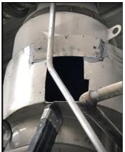
Then we applied Belzona 1111 Next we applied the first plate for the adhesion of the plate using Belzona 1111.
