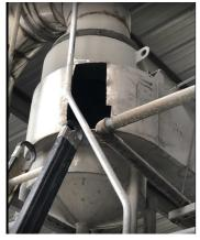
The first picture is where the granules had eaten away the surface of the cyclone. We had to cut it out to make it a better sealing surface.
