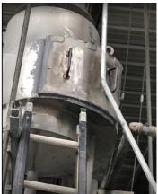
Then we applied the final piece that was custom made for this application. (Note the handles) This piece was really heavy due to the material it was made from and the added weight of Belzona. But this allowed for removal and touch up for future use.
