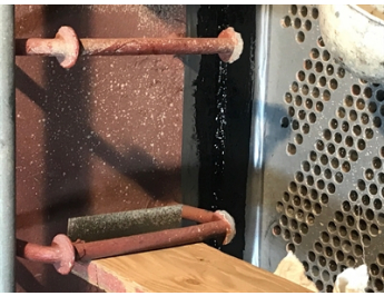
Closeup of Belzona 2111 elastomer expansion joint in main condenser
