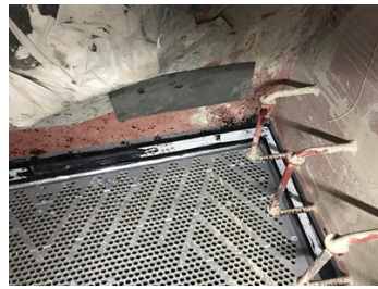
Belzona 2111 application reinforced with reinforcement mesh replacing expansion joint
