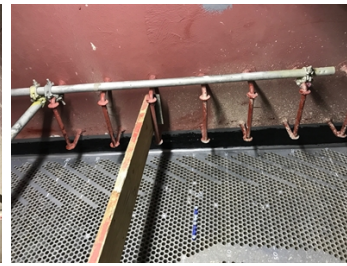
Close-up of final expansion joint using Belzona 2111 elastomer
