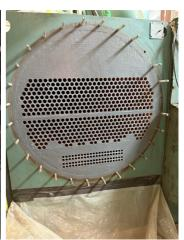
Severe corrosion present on the tube sheet of the YORK MaxE chiller, showing metal loss, scaling, and deterioration around the tube openings prior to surface preparation.
