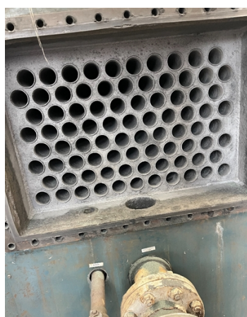
After abrasive blasting SSPC-SP10
