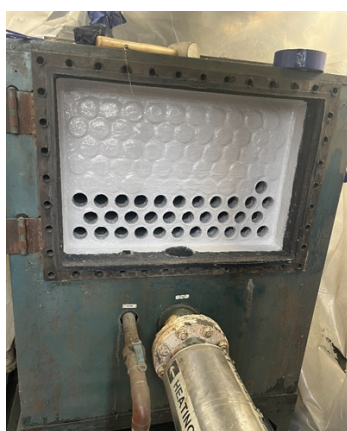
Pit fill and first coat applied of 1391T. Corks still in place.
