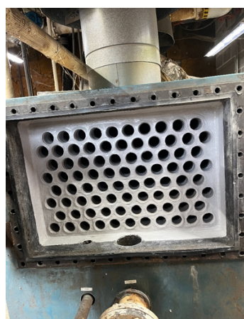
Corks removed and final touch ups completed.
