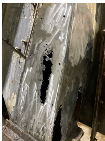
Surface prep complete with power tools.
