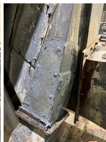
Plate bond application.
