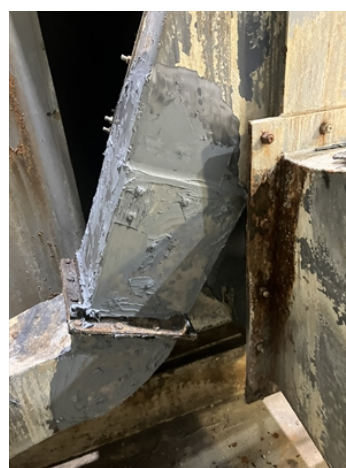
Plate bond application.
